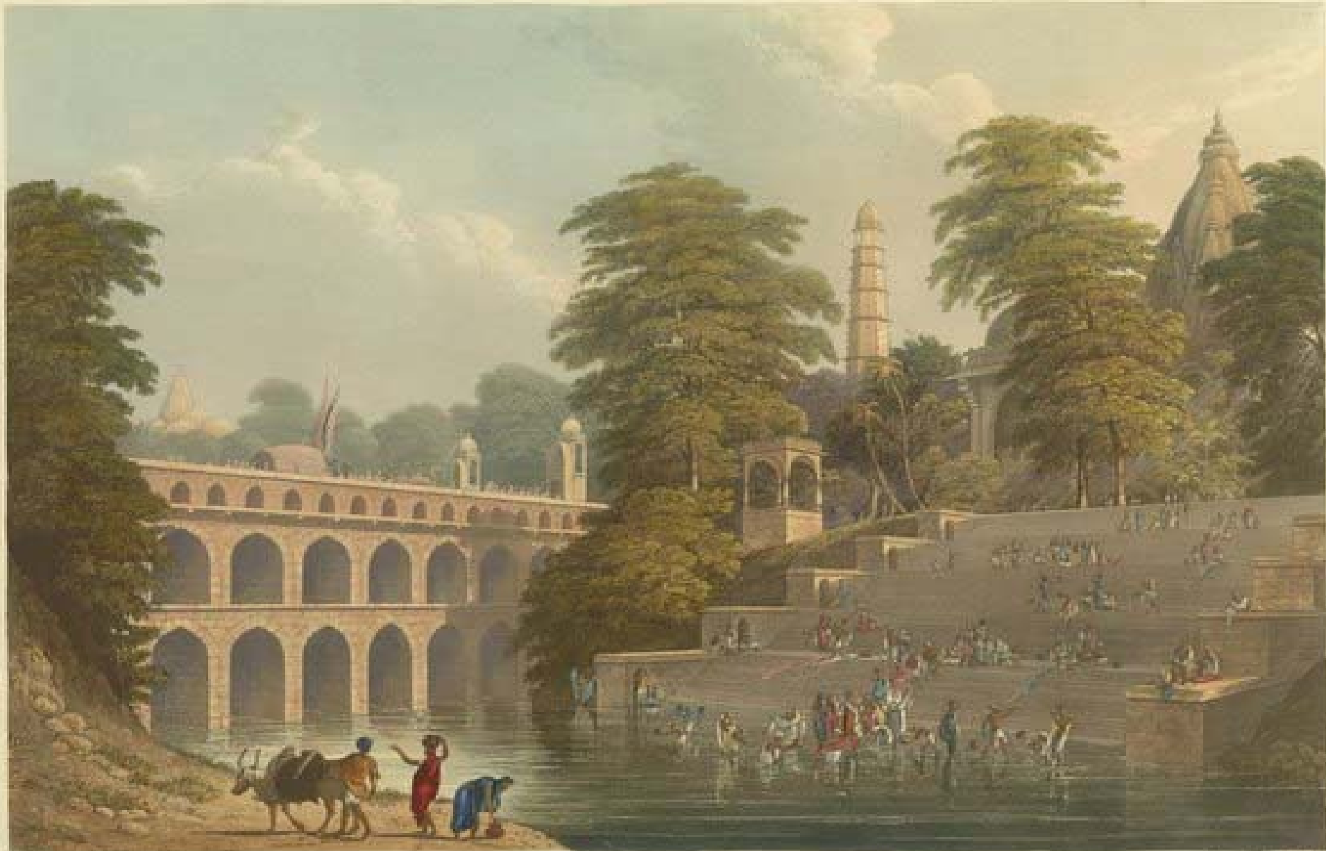
View of the Bridge near Baroda in Gujarat.
